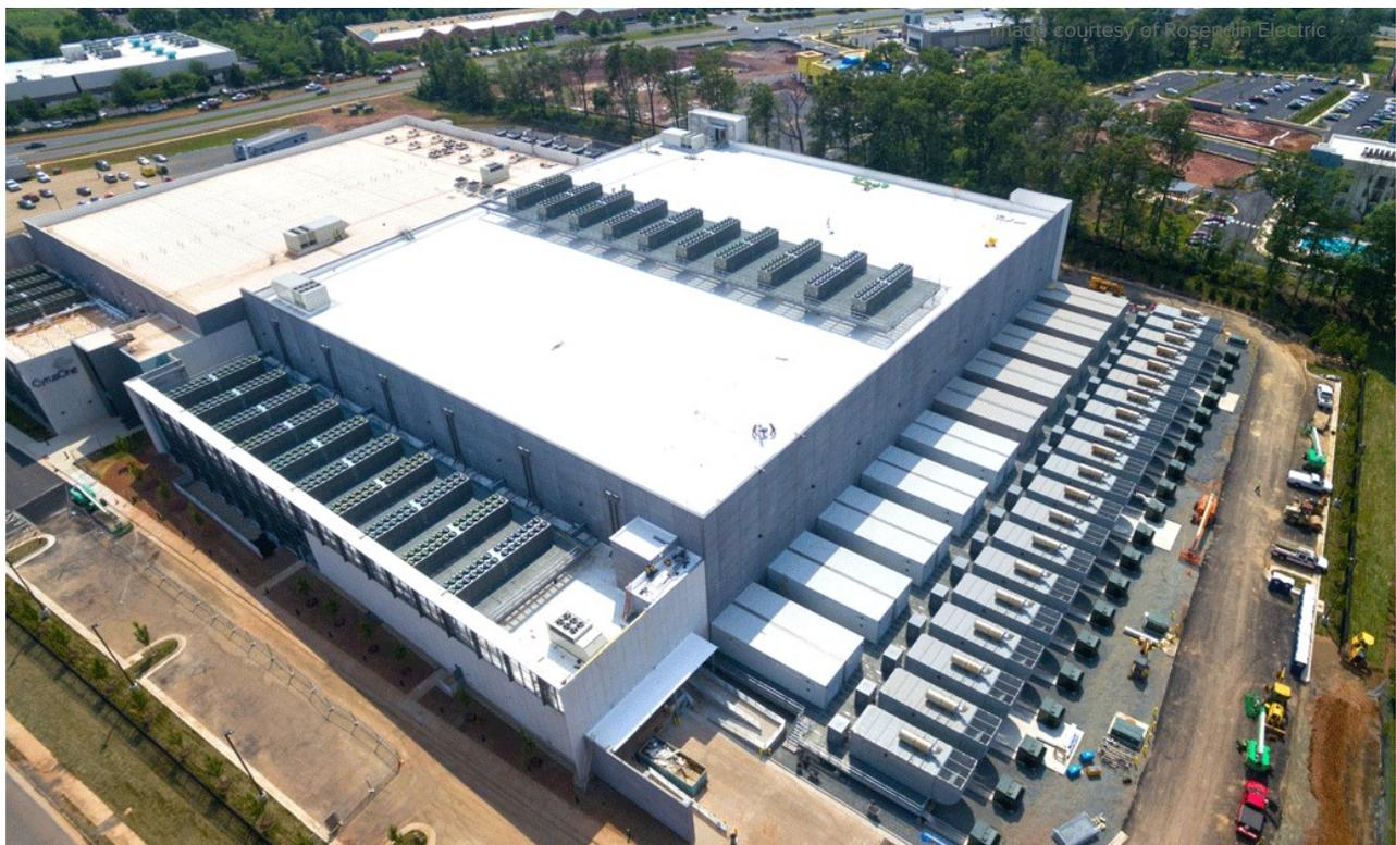
This 220,000-square-foot data center, nicknamed Project Goliath, included twenty 2,500kW generators and was completed for an enterprise client in less than six months.
